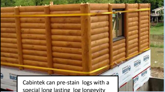
To save time simply install the windows as you are installing wall logs. Windows install in minutes
