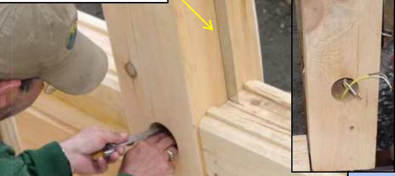
Each vertical log has a 4" hole that is used to thread the nut on the anchor rod and also the hole becomes an opening for an electrical base outlet
