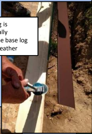
Factory pre-cut log starter plate is positioned over the anchor bolts and raises the base log to create a wiring chase so wiring can be installed after the cabin is up
