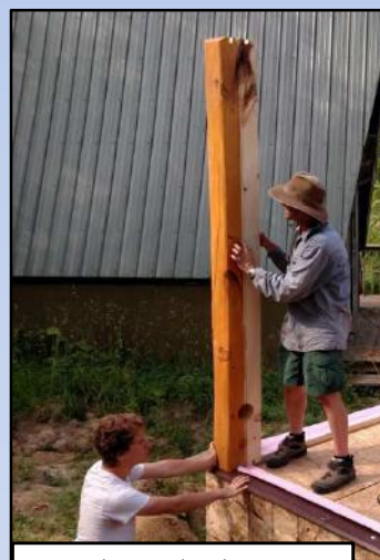
Vertical corner log- being placed and braced
